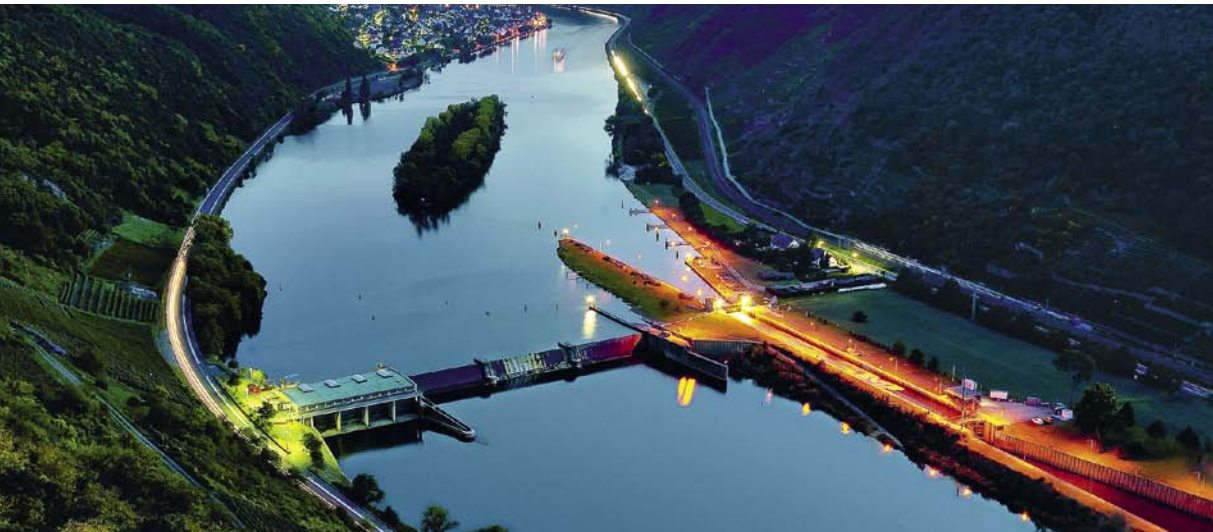
The growth market of rail freight transport benefits from rail's environmental advantage and the ongoing liberalisation of the rail markets (far left: hydroelectric power station on the River Moselle which will supply electricity to DB as from 2014).
